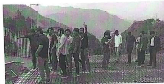
Students inspecting R/F of the Bridge Deck
